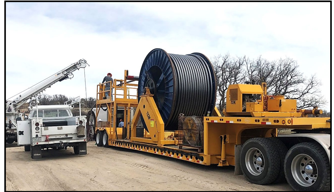
Underground Reel on Custom Trailer for Cable Pulling
