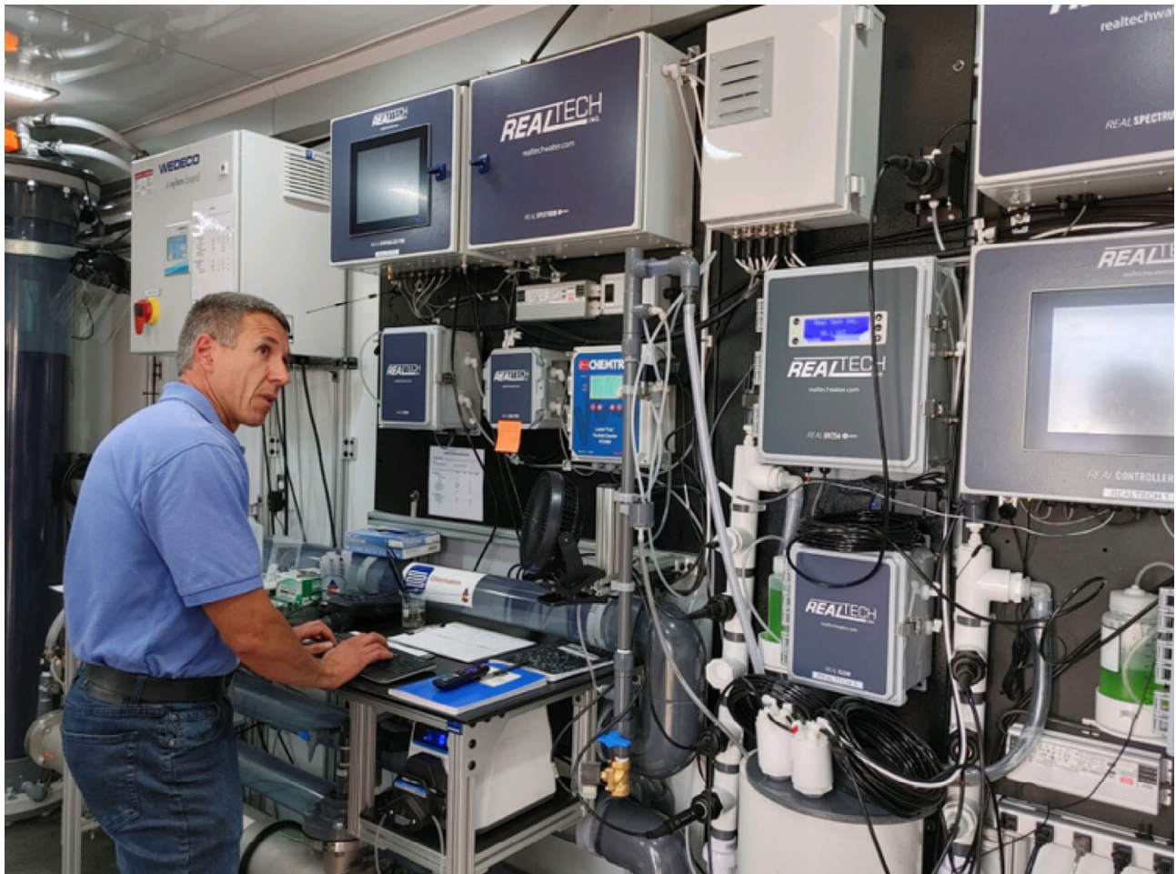
Utilities' Kirk Olds checks the readings inside the mobile unit that turns treated sewage water into drinkable water.
