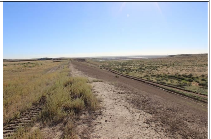
Photo #34 Facing East
