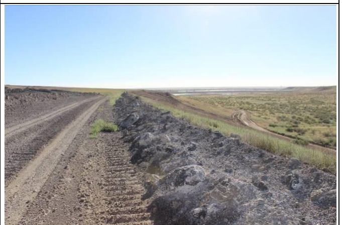
Photo #36 Facing East
