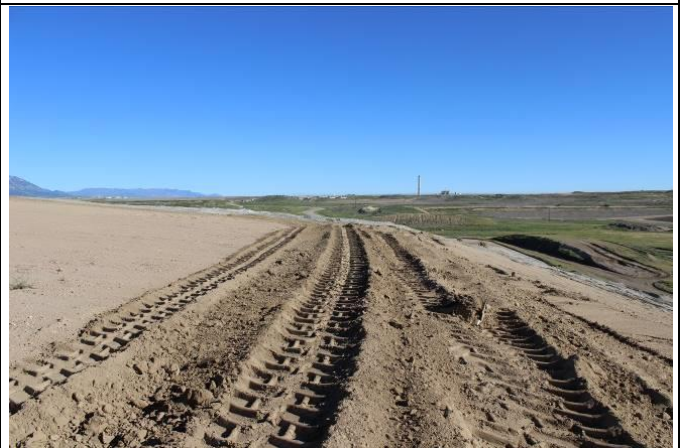
Photo #40 Facing North
