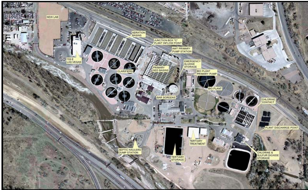
Figure 1-2 Las Vegas Street Water Resource Recovery Facility
