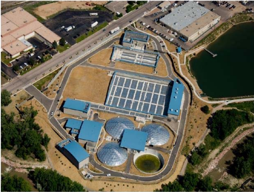
Figure 4-8 J.D. Phillips Water Resource Recovery Facility
