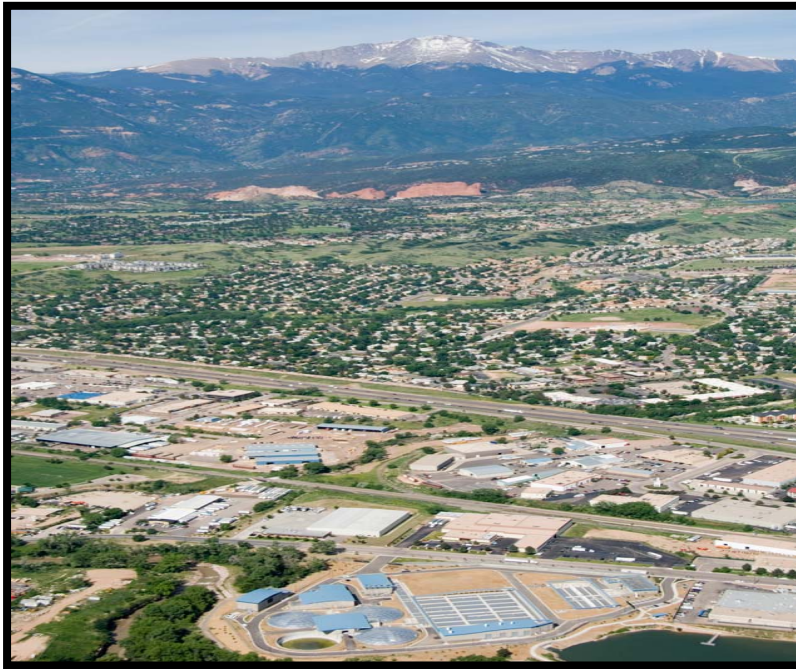
Figure 1-1 J.D. Phillips Water Resource Recovery Facility
