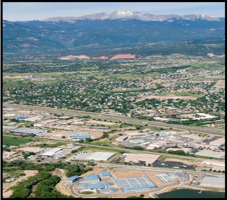
Figure 4-7 J.D. Phillips Water Resource Recovery Facility
