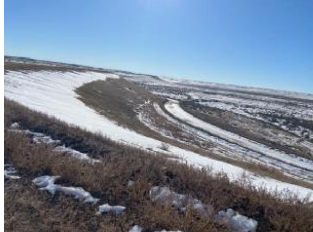
Photo No. 20, 11.13.2024 Observations
