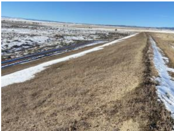
Photo No. 17, 11.13.2024 Observations
