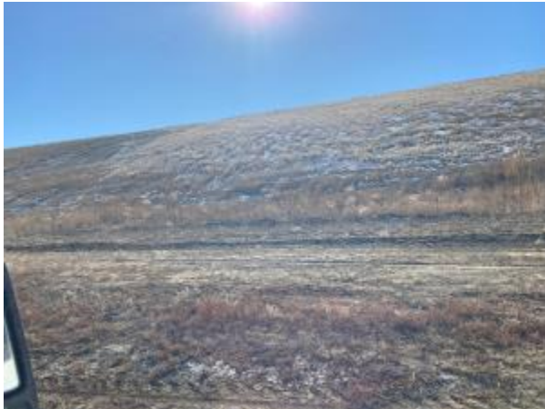
Photo No. 48, 12.03.2024 Observations
