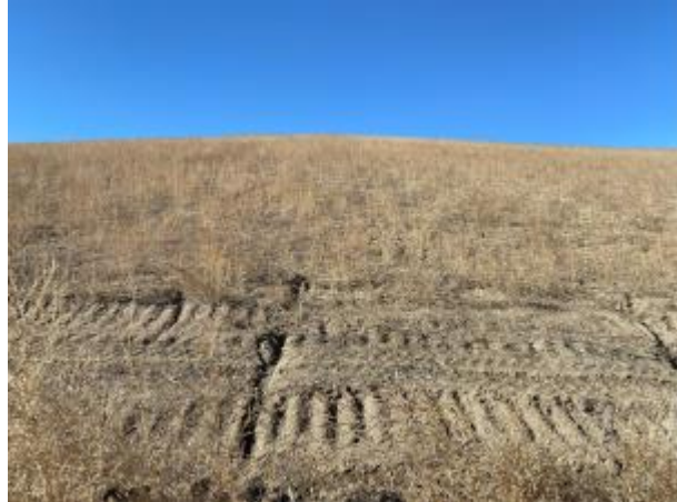
Photo No. 35, 12.03.2024 Observations
