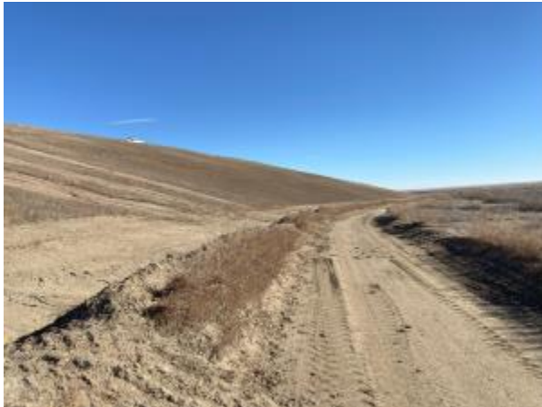
Photo No. 30, 12.03.2024 Observations
