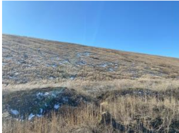
Photo No. 43, 12.03.2024 Observations
