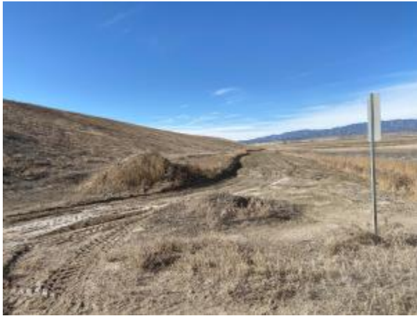
Photo No. 50, 12.17.2024 Observations
