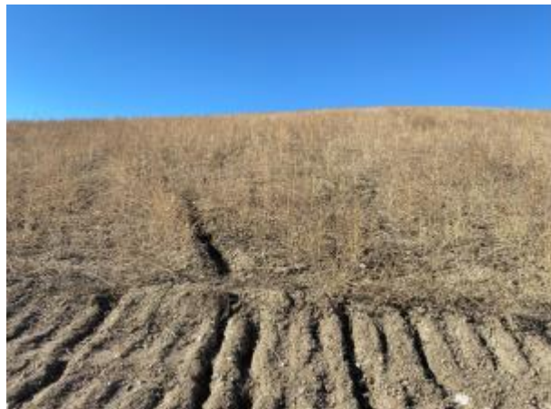
Photo No. 39, 12.03.2024 Observations
