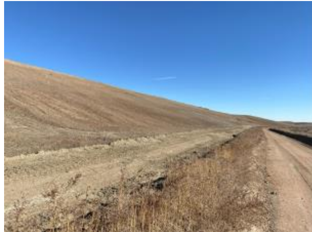
Photo No. 25, 12.03.2024 Observations
