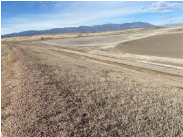
Photo No. 58, 12.17.2024 Observations
