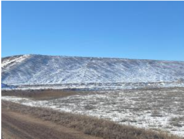
Photo No. 1, 11.13.24 Observations
