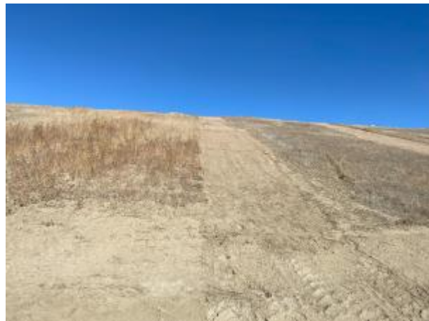
Photo No. 27, 12.03.2024 Observations
