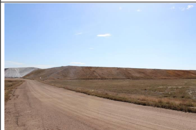
Photo #41 Facing Southwest
