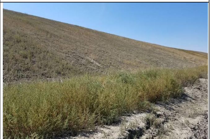
Photo #36 Facing Southwest
