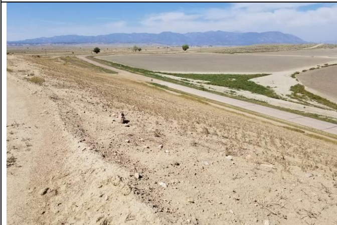
Photo #33 Facing Northwest
