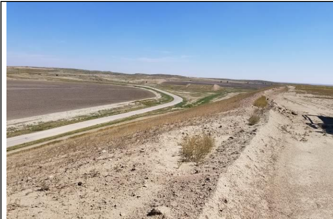
Photo #31 Facing Northeast
