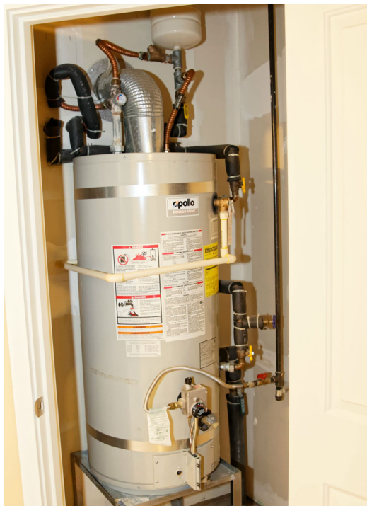
ENERGY STAR® gas storage water heaters use about 10% less energy compared to standard gas water heaters.
