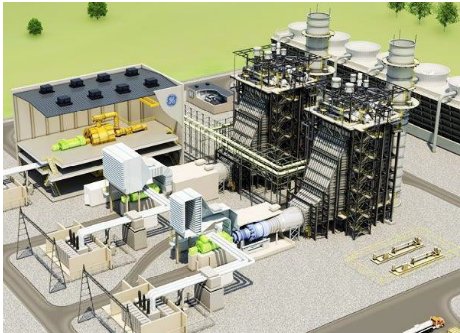
Figure 4-8: Combined Cycle Power Plant Layout
