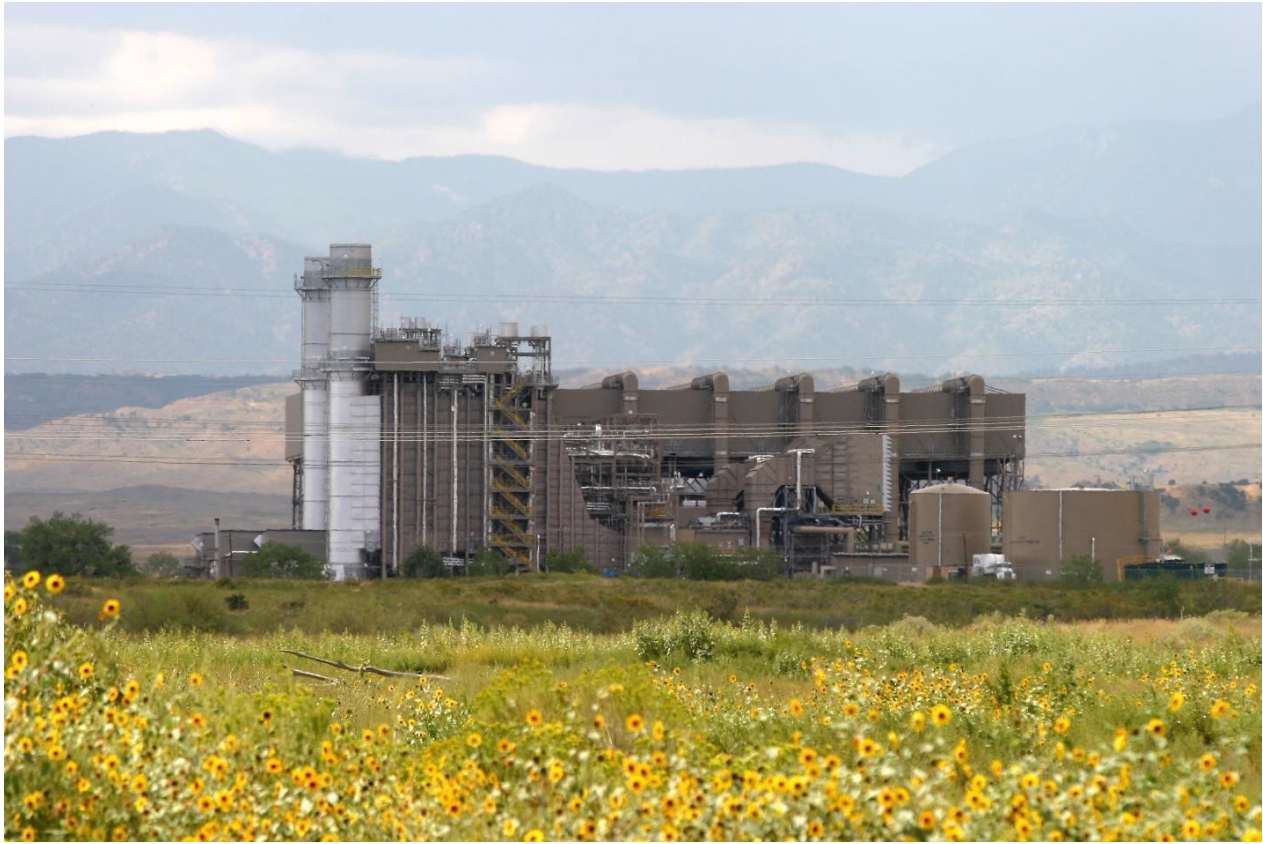
Figure 3-3: Front Range Power Plant
